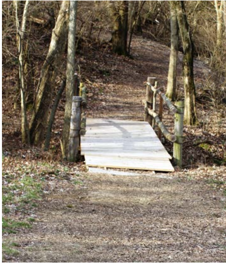
Bridge over creek
