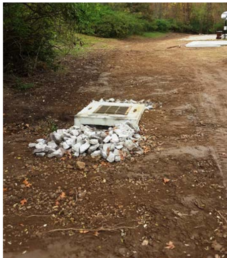
Carmack Park Pipe Replacement
