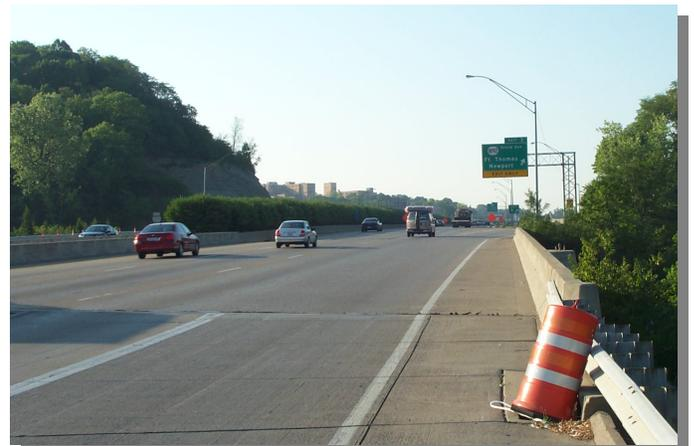
*Existing shoulders on I-471 are not suitable for bus travel due to narrowness and insufficient structural capability to handle continuous traffic.*
