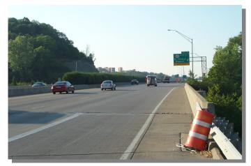
Existing shoulders on I-471 are not suitable for bus travel due to narrowness and insufficient structural capability to handle continuous traffic.
