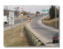
Ramp metering has been successfully employed in over 4,000 U.S. locations, including the Columbus, Ohio location depicted here.
